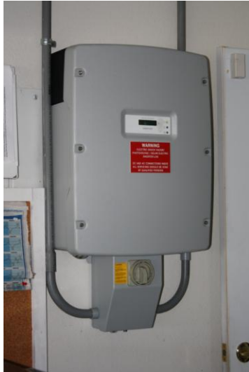
Figure 8 – Inverter
